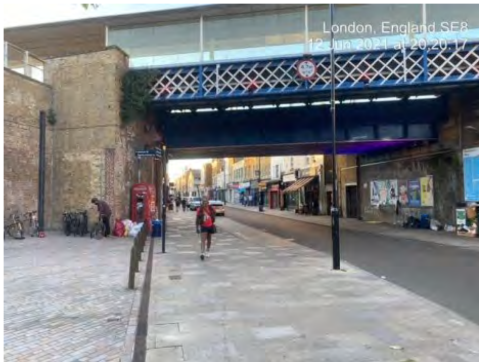
Image A22 Looking north at Deptford Rail Station - 20:20hrs
